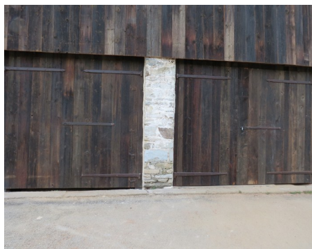
Above: New barn doors and hinges.
